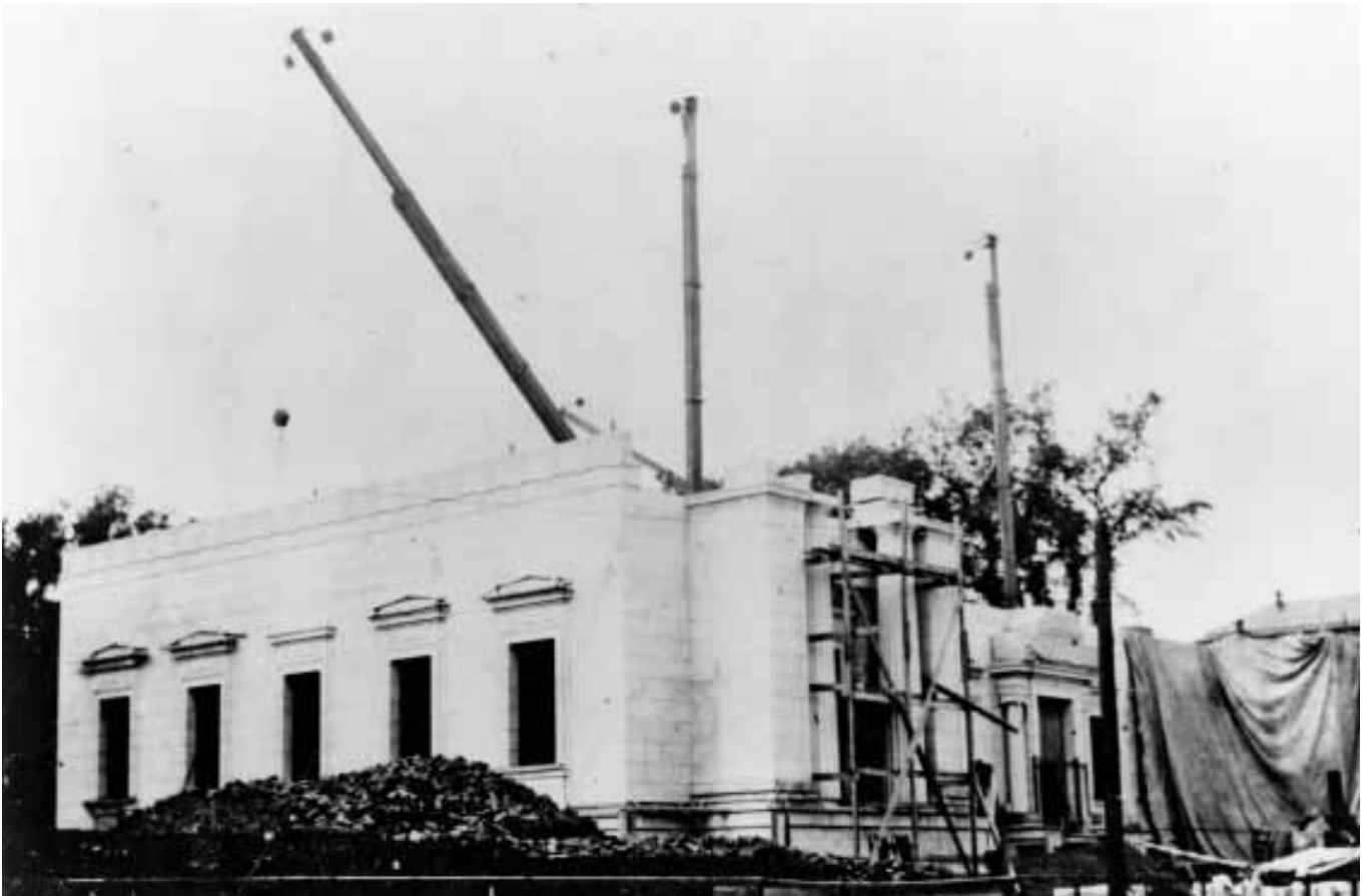
Work on hold for the winter, 1909–10. Progress during the fall was slow, and, despite warnings from Lowell, the roof was not capped before cold weather arrived. In the spring the tarpaulins were thrown aside, and the walls again began to rise toward the cornice. Rough blocks of granite appear over the doorway where the sculptural group is today. New Hampshire Historical Society.
